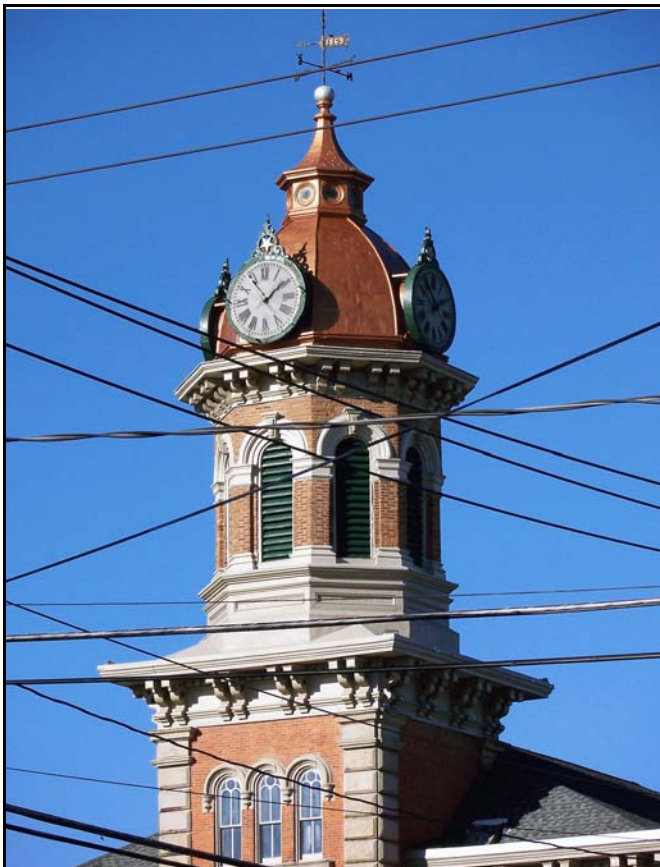
Someone got their wires crossed
